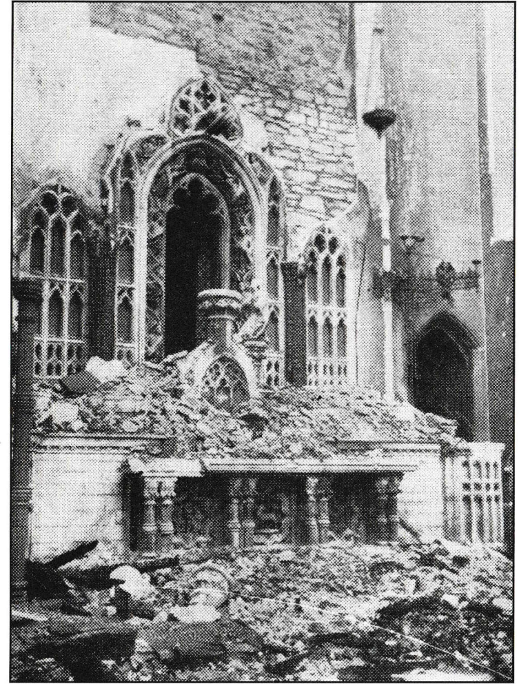
The high altar was destroyed by enemy bombing on the night of 3rd March 1941. It was to lay derelict for eighteen years.
